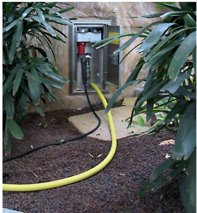
Water Park Rheinwelle, Gau-Algesheim, Germany
